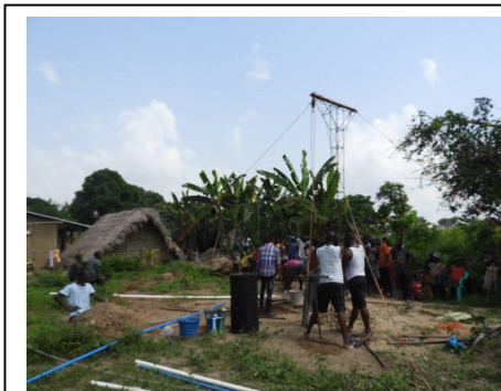
Figure 8 Drilling in Sembehun
